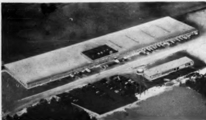
Airview of Winn-Dixie's Greenville, S. C. warehouse, one of the South's largest and most modern food distributing facilities.
